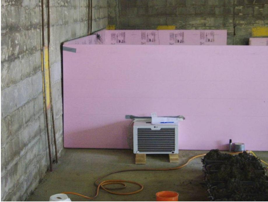
FIGURE 4. AIR CONDITIONING UNIT INSTALLED IN STYROFOAM ENCLOSURE
